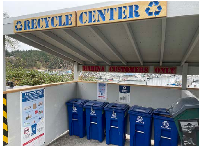
Port-Built New Recycling Center
